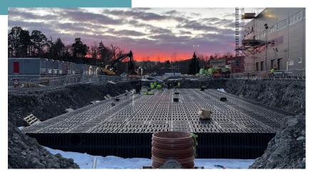
Attenuation = Membrane to be adapted in combination with geotextiles for protection it acc.
